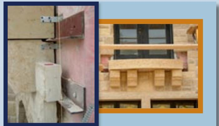
A plumb line stages the offset of the surrounding veneer as it finishes out the window sill.
