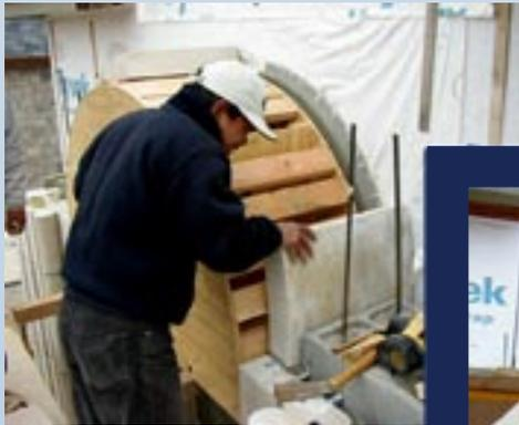
Wooden forms are used to support the stone as it is being fitted and placed.
