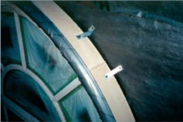
Note the protective tape covering the stone face, which will prevent any mortar spillage from staining the stone pieces.
