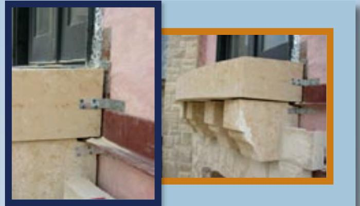
L-Clips & Tapcon screws secure the stone in position. Steel beams support and distribute the weight
