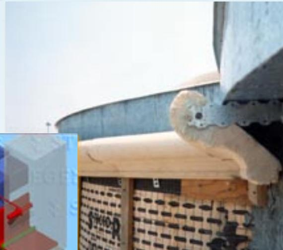
Supporting the weight from below is the main goal and preventing the stone from "rolling away" from the structure.
