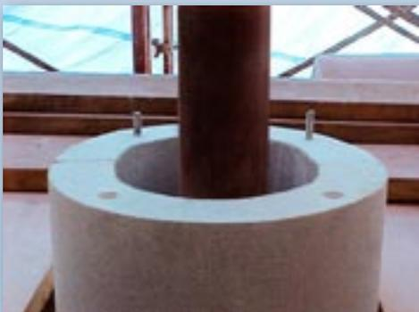
Precast holes are set with pins to align the column sections
