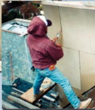
Filling mortar gaps and smoothing with a pointer
