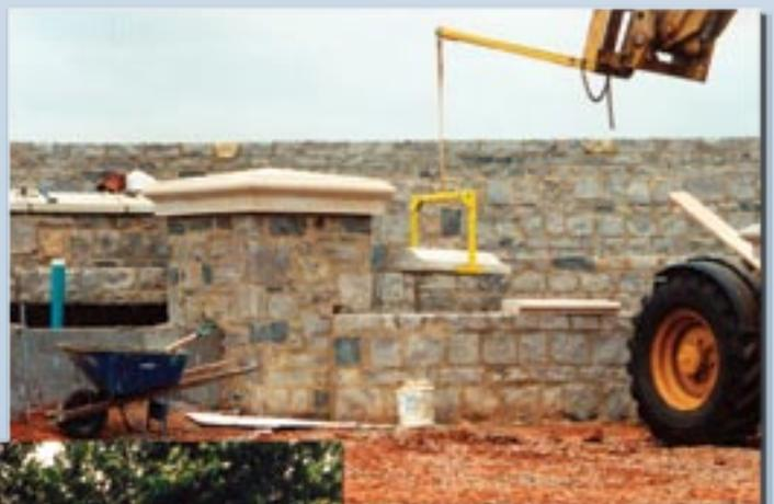
A hoist crane is used to lift & place heavier stones
